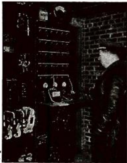
Control panel for the new U.S. Navy blind-landing system. Current supplied by a 500-cycle motor-generator is fed through this panel to the buried cables which set up the magnetic beam (which has a range of 9,000 ft.).
